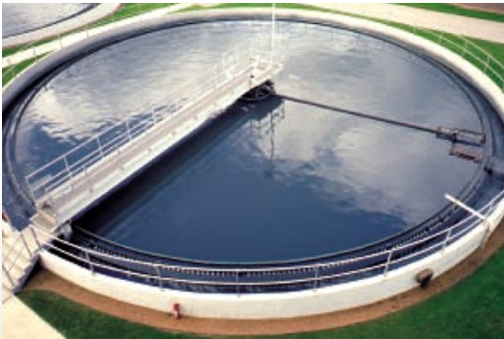
BayWork Activated Sludge Overview 2021
