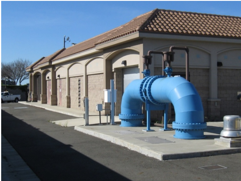
Skywest Pump Station
