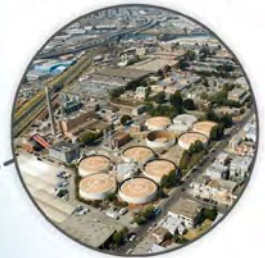
SOUTHEAST TREATMENT PLANT
