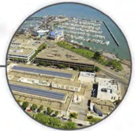
NORTH POINT WET-WEATHER FACILITY
