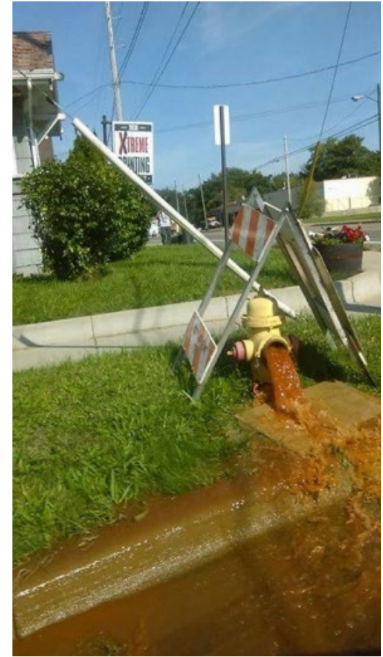
Photo credit: Erin Brockovich of actual Flint flushing
