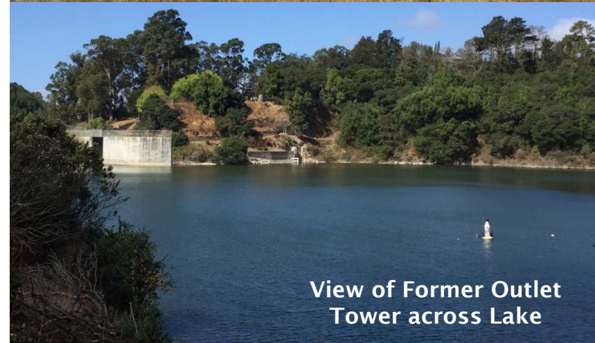
Final Downstream Slope of Dam
