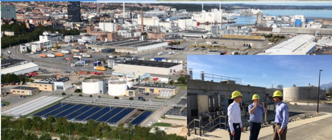
Wastewater & Energy Neutrality
