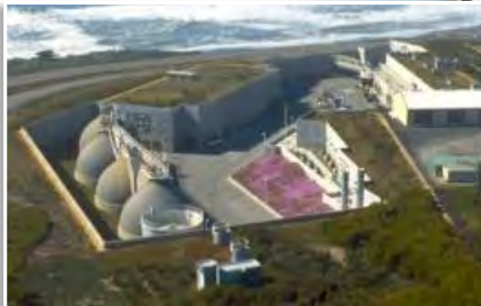
Oceanside Treatment Plant
