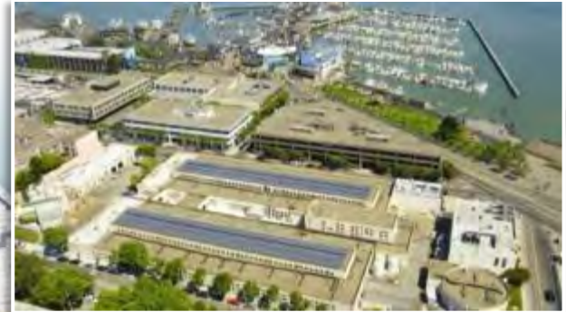
North Point Wet Weather Facility
