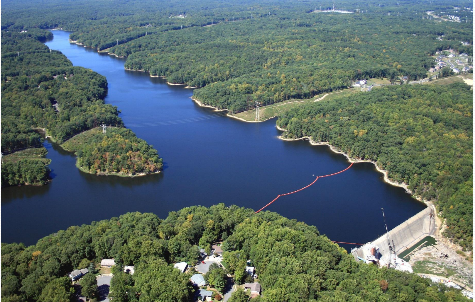
Photo Courtesy of Roger Snyder Virginia Tech, UOSA, Occoquan Reservoir
