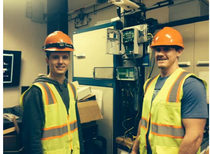
Figure 5.2: Los Medanos College instrument and control technician interns working at
