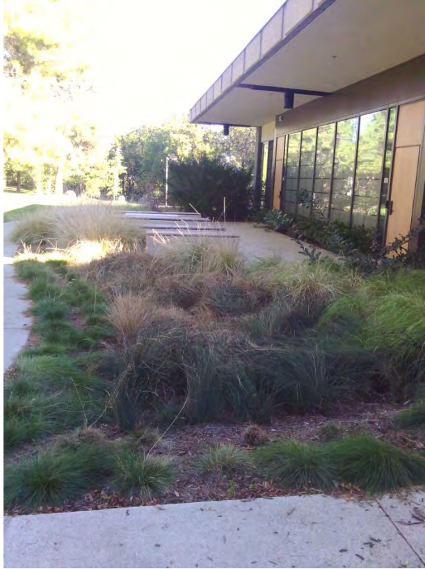
Bioswale in front of LA/SS building-side view. Photo Credit: Corey Chetcuti
