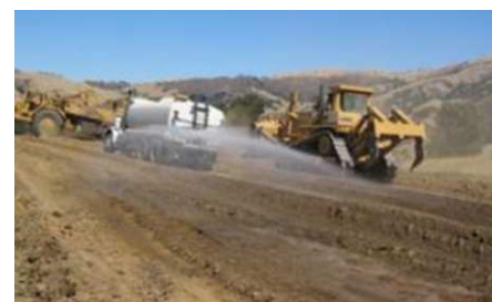
Above: Water truck provides dust mitigation by wetting road surface.
