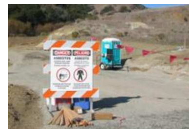
Below: Restricted area danger sign displays the required PPE with orange flagging to restrict entry.
