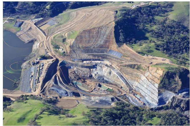
View of Calaveras Dam Site (from right side of valley)
