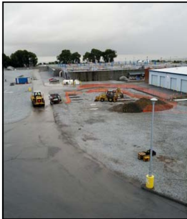
Potholing and Locating Piles
