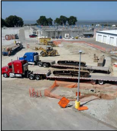
Pile Driving Equipment
